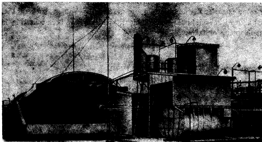
FIG. 64. Nitration Biazzi system building surrounded by earth mound with service tanks in centre and right foreground. The nitration building is protected by lightning arrestors [47]. (I.C.I. of Australia and New Zealand Ltd. at Deer Park, Victoria).
