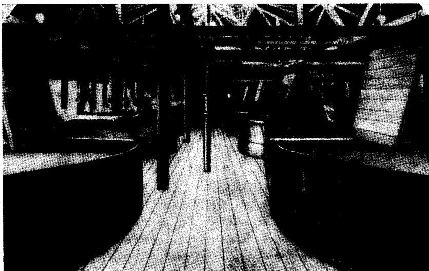
FIG. 152. General view of digesters for stabilization of nitrocellulose (Hercules Powder Co., [3]).
