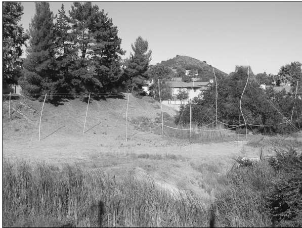
Figure 6-6: Story poles are required in some cases to let neighbors know how your house will affect sight lines and aesthetics.
