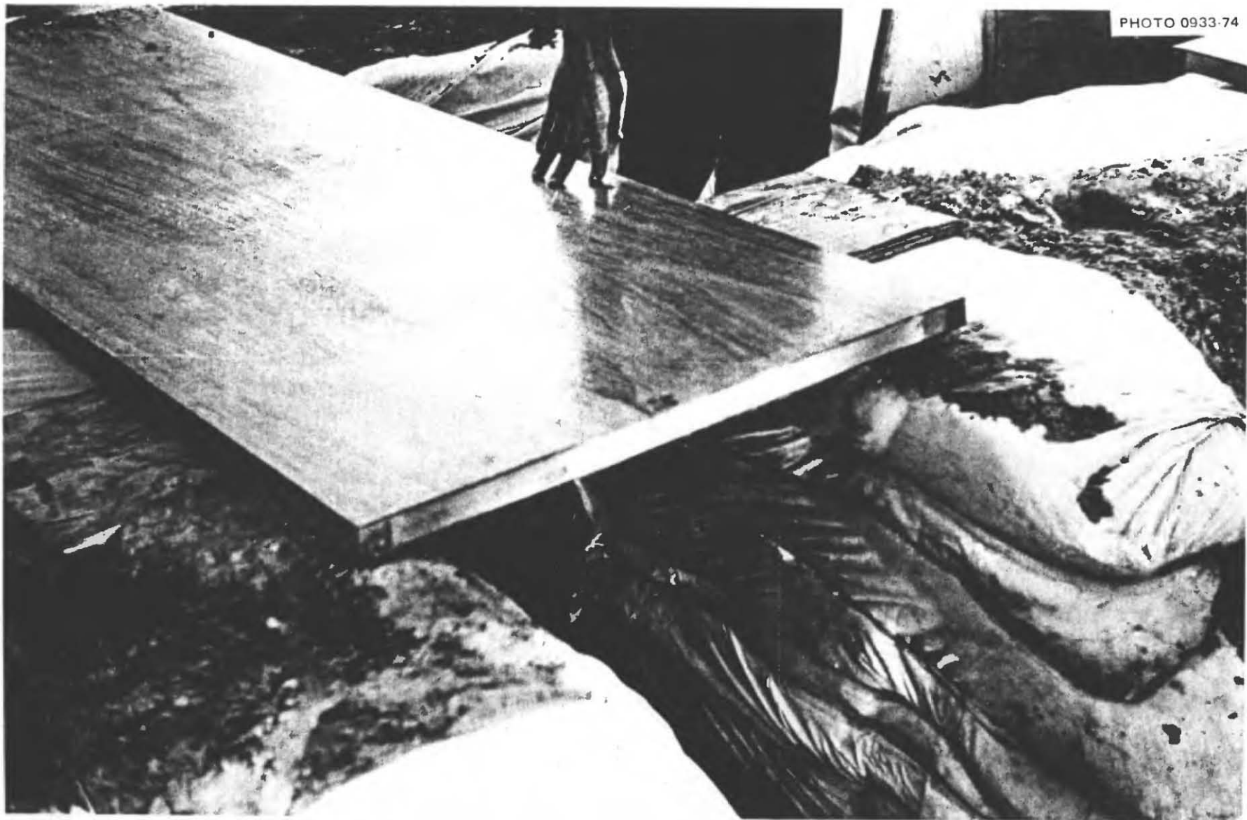
Fig. 5.8. Placing an interior door over one end of the shelter and part of an entryway. The wall of this entryway consisted of 7 small rolls which were made by using pieces of sheets and other cloth, with the outer ends tucked in.
