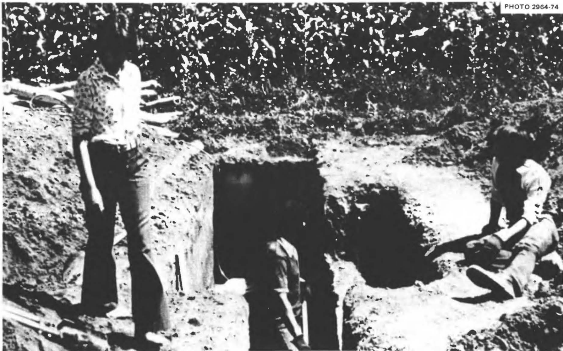
Fig. 4.5. The small ledgelike excavation on the side of the main trench was dug by Kearny to provide himself with a place to sleep and to observe the shelter-occupancy test. This sleeping ledge was 2 \times 8 ft, providing a height to the log roof of only 2 ft. After Kearny got a sore neck from turning around periodically on this sleeping ledge, with only a 24-in. ceiling, during the 77 hours of shelter occupancy, he concluded that such sleeping ledges should be dug to provide a 30-in. ceiling.
