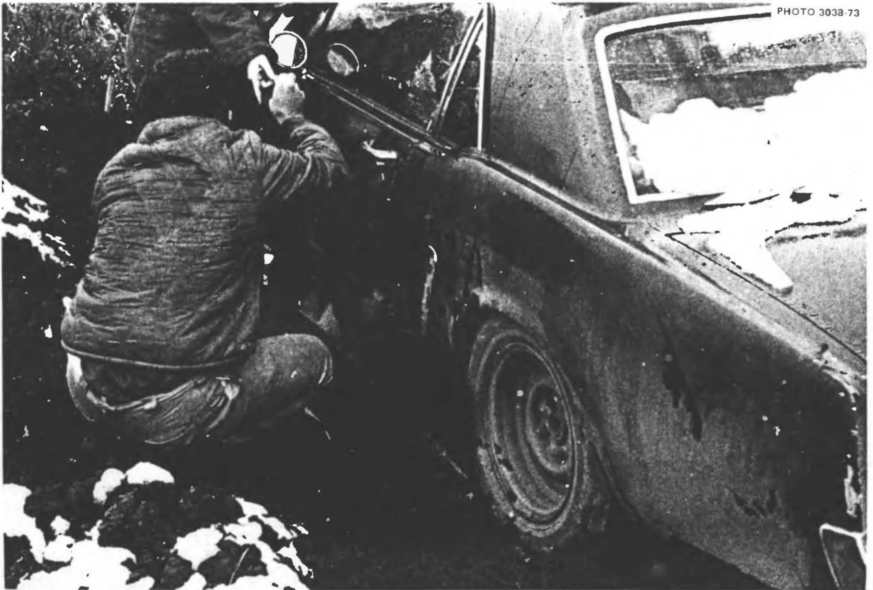
Fig. 6.12. Taping split-open plastic garbage bags to the sides of the car, for want of other waterproof material to keep some of the dry earth to be mounded around the car from running under the car onto the storage "shelf" areas around the edges of the trench, or into the trench. Fortunately, the father had some waterproof duct tape, and cleaned the dirt off the spots on the car to which he planned to tape the plastic. However, because he did not tape all of the upper edges of the pieces of plastic, if water had run down the sides of the car, much of it would have run under the upper edges of the plastic and into the shelter space under the car.
