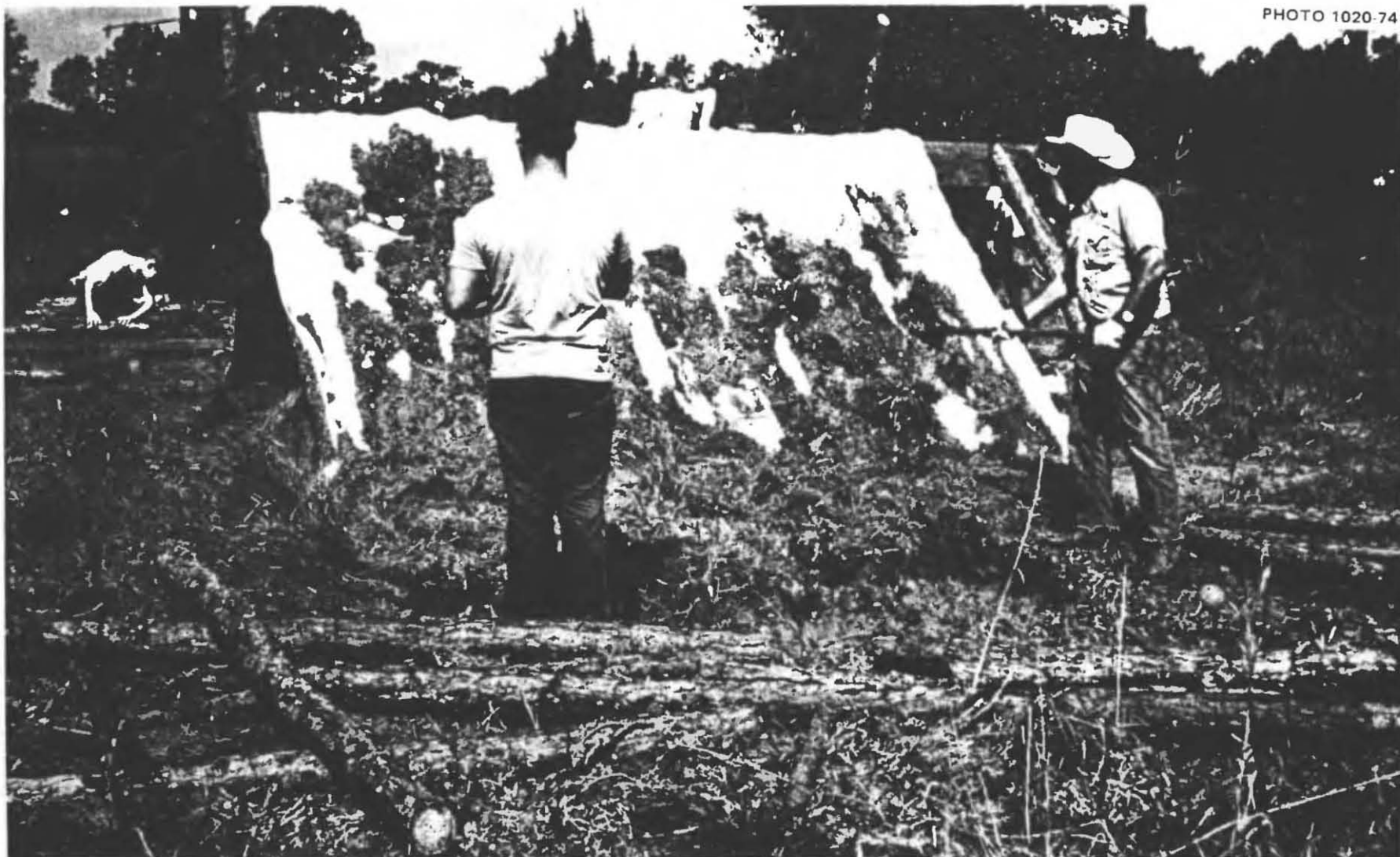
Fig. 5.47. Starting to cover part of the completed side walls with earth. Since these families had plenty of sheets and bedspreads, they placed some directly on the wall poles to keep sand from falling through the cracks.
