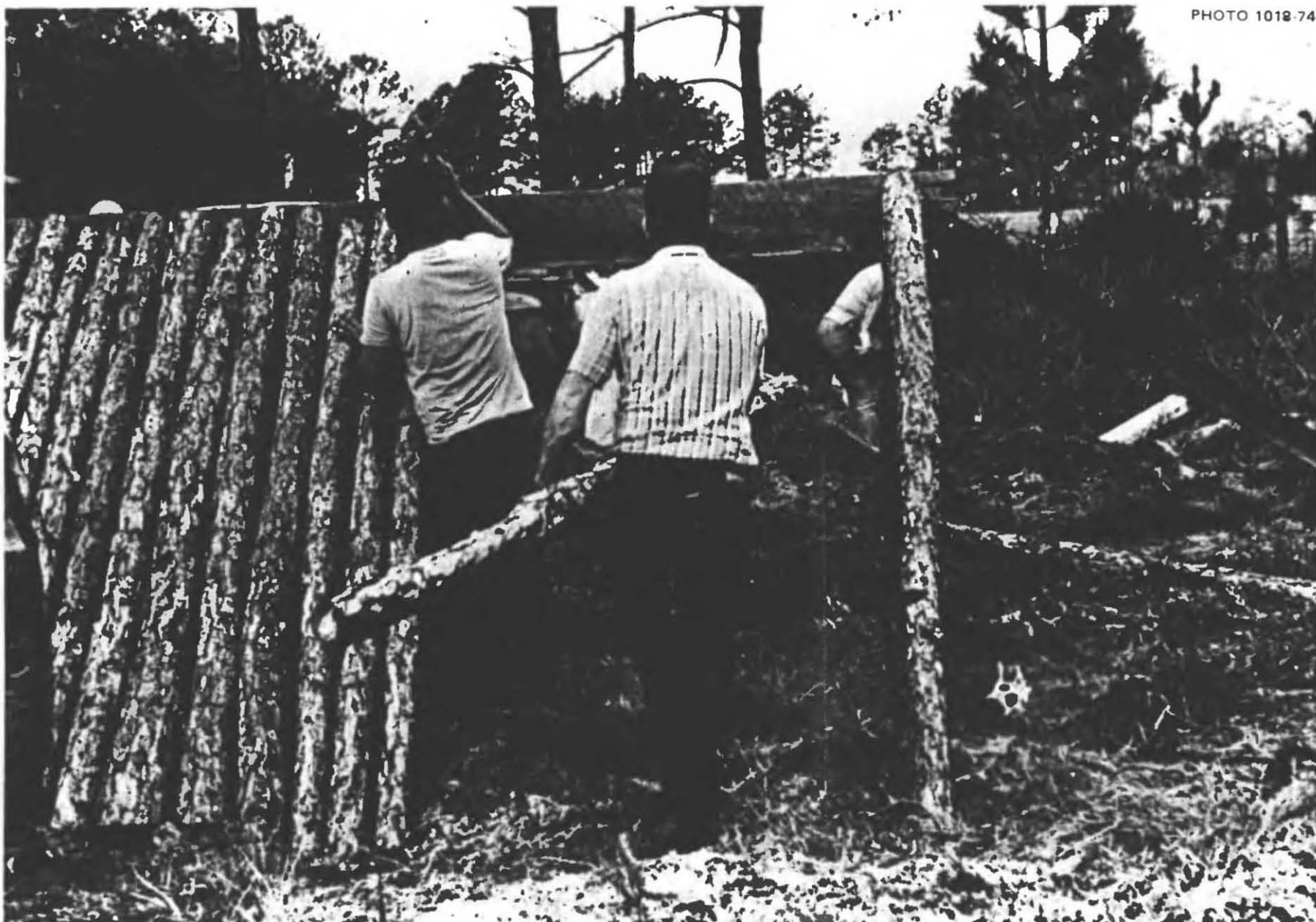
Fig. 5.46. Nailing a 9-ft roof pole to the ridge board. This photograph is misleading as regards the lower ends of the ridge poles; actually the ends rested against a 1 × 6 board placed against the outer side of the 6-in.-deep V trench that marked the edge of each shelter side wall.
