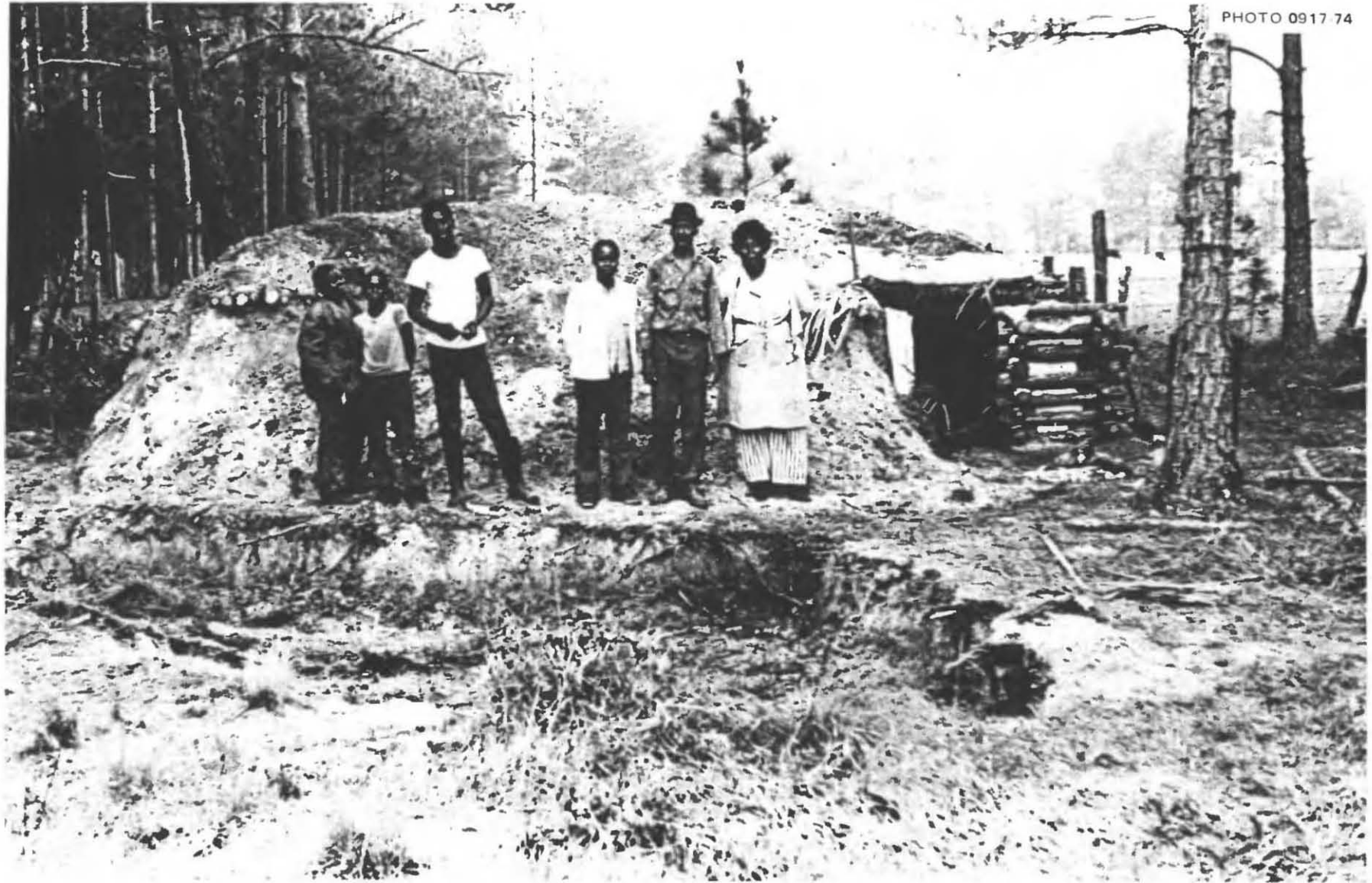
Fig. 5.24. The successful builders outside their completed shelter, with a full 2 ft of earth on the roof. Note one of the shallow barrow pits, from which they had shoveled and carried earth, in buckets and a wheelbarrow, to the adjacent building site.
