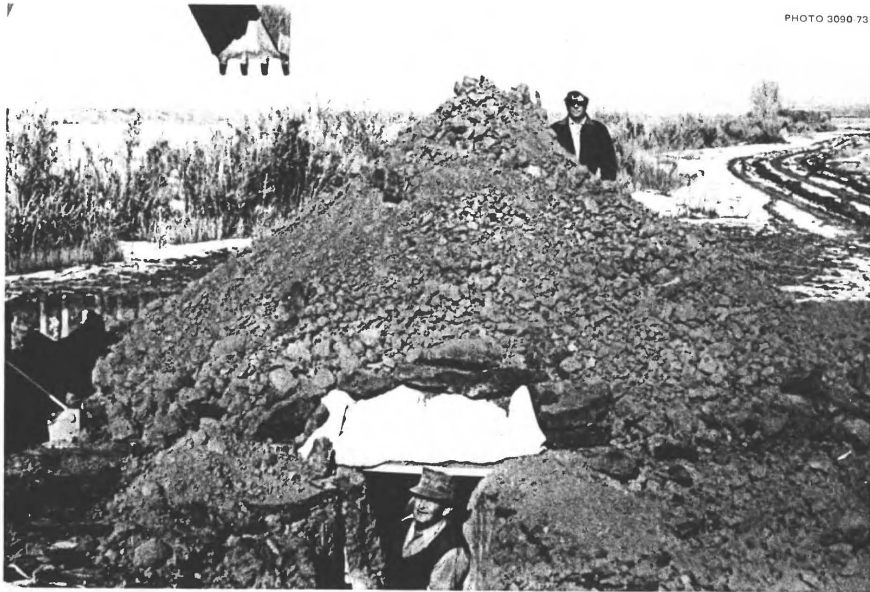
Fig. 3.2. View of the same shelter from the entryway end. An observation trench had been dug out from the entryway, so that deflections of the roof doors could be observed safely.
