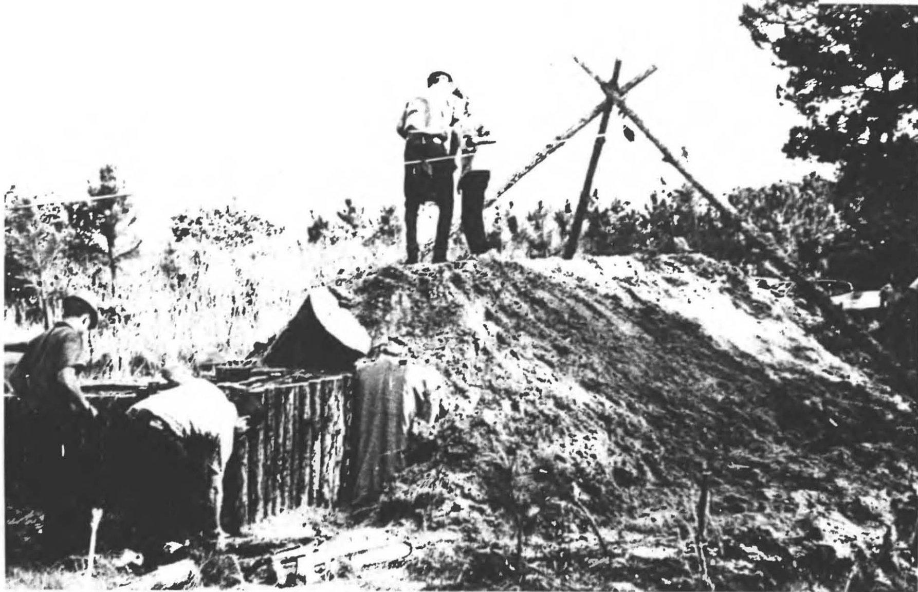
Fig. 5.51. The pulley conveyor system actually wasted energy and time, since earth had to be lifted in a 5-gallon paint can up to the hook on the movable pulley; then the earth-filled can was pushed up the upward-sloping nylon rope to a position several feet above the top of the shelter. Then most of the earth rolled down below the top of the shelter, obviously wasting thousands of foot-pounds of work.
