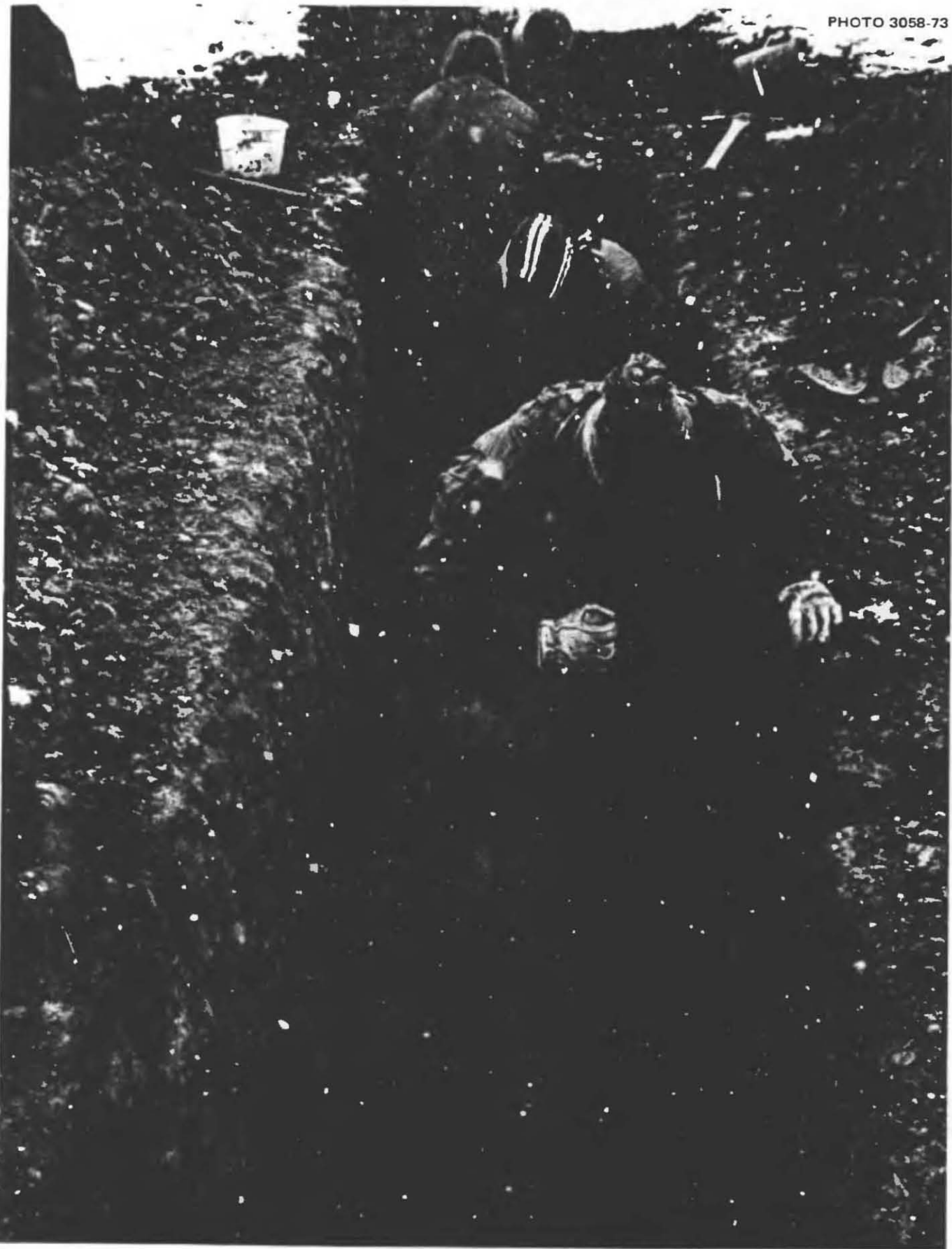
Fig. 2.7. At 8 AM on the second day, when the trench was about 3 ft deep, this family had the good fortune to get below the dry, hard clay-loam and into a slightly sandy clay-loam. The mother could dig this very stable but not-so-hard earth by standing on the shovel and slicing and prying off rows of chunks from the edge of a 6-in.-high earth step.
