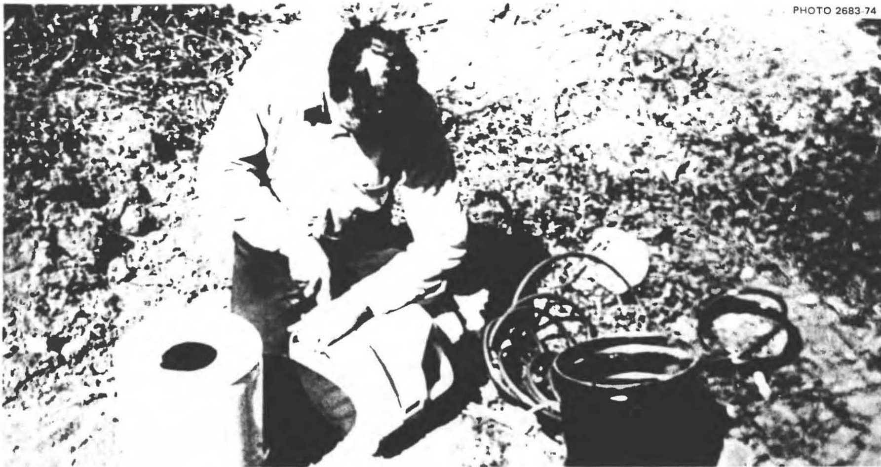
Fig. 4.26. Using a sharp knife to cut off the lower part of the 5-gallon plastic water jug, in order to make the bowl of the toilet. The bottom of the 5-gallon can shown on the right was cut out so that when this can was used to form the bottom of the 10-gallon vented space provided for the wastes, the liquid fraction could run into permeable earth or sand below.
