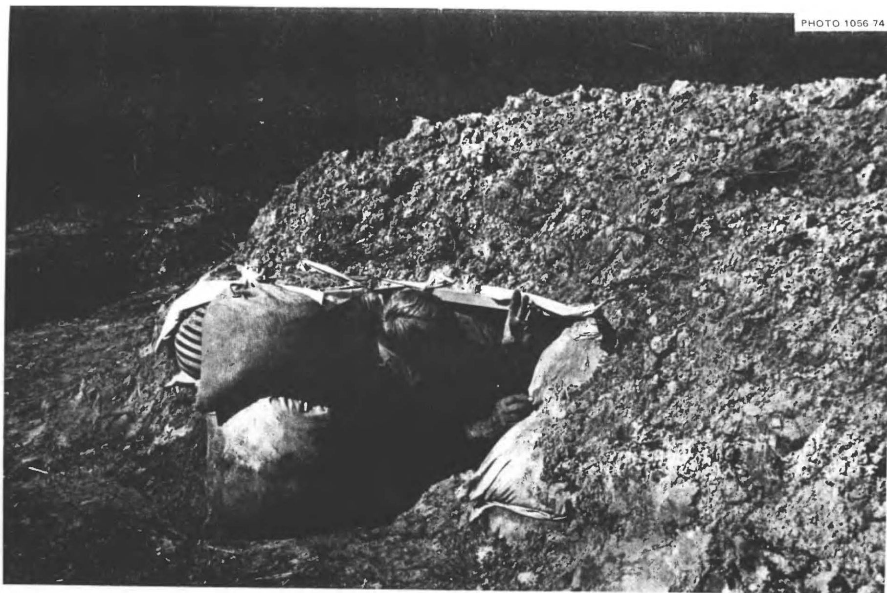
Fig. 5.10. A closeup view of the same entry pictured previously, showing the sandbags used to finish the ends of the entryway walls and to reduce radiation from fallout on the ground, which otherwise would enter the shelter.
