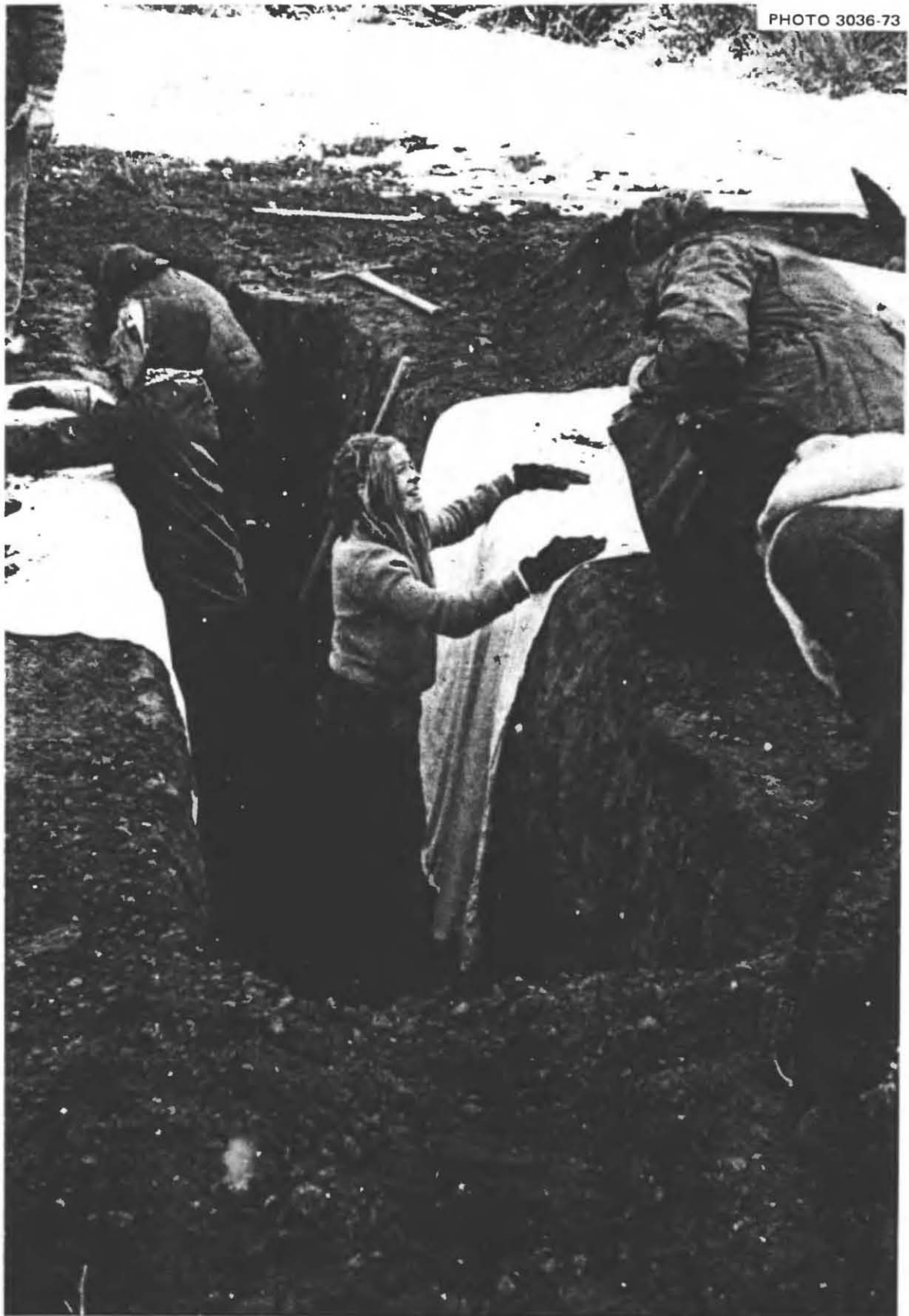
Fig. 2.8. Placing bedsheet coverings on the 4\frac{1}{2} -ft-high trench walls. Such coverings make the trench cleaner, warmer, and easier to illuminate.
