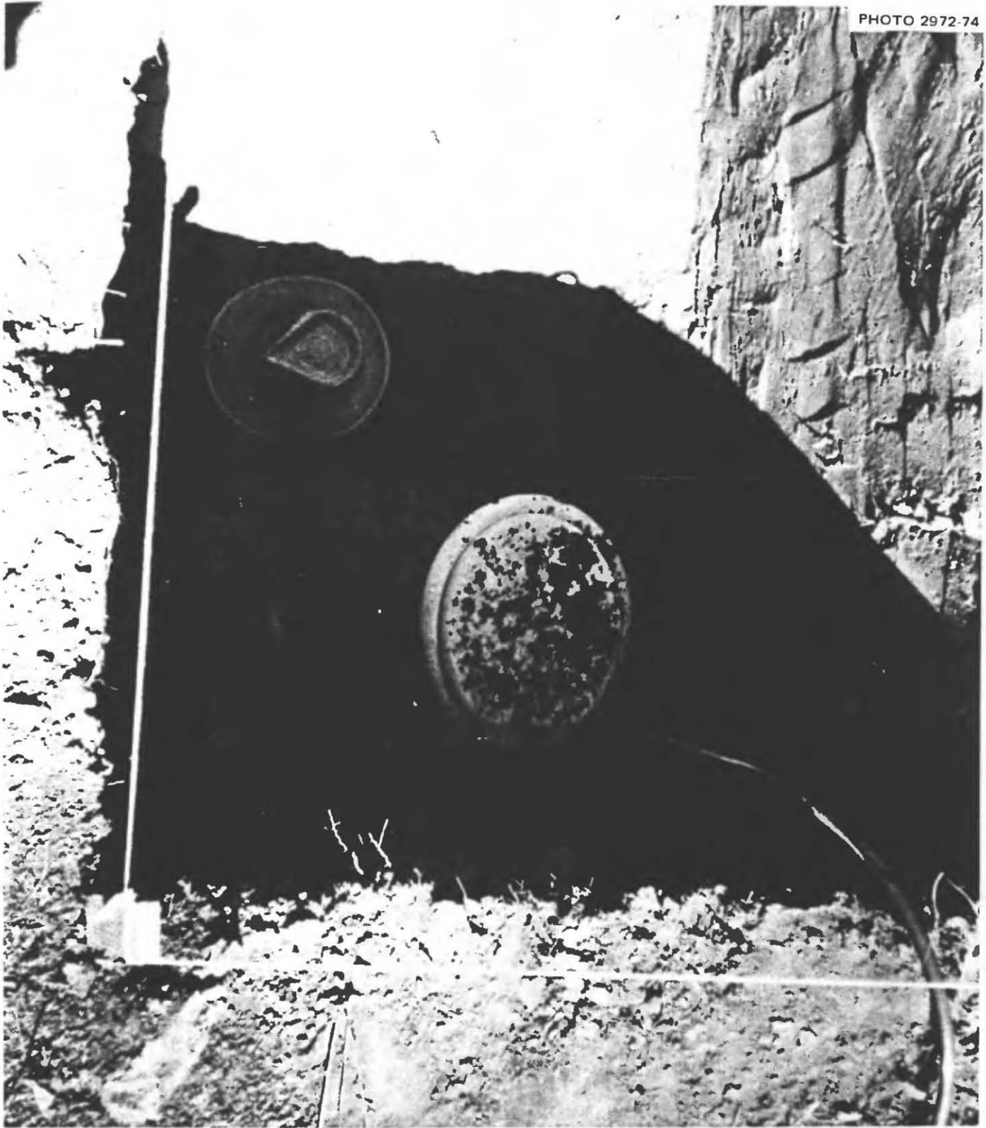
Fig. 4.29. View looking straight down on the installed toilet and its seat. The two assembled 5-gallon cans and the toilet bowl had been placed in a hole dug in the bottom of the shelter. A piece of \frac{1}{2} -in. plywood, in length equal to the 42-in. width of the shelter room and about 20 in. wide, served as the horizontal surface to which the toilet seat was attached. An appropriately sized, roughly elliptical hole had been cut in this plywood with a brace and bit and a cold chisel. The plywood base of the toilet was at floor level. Note the vent hose.
