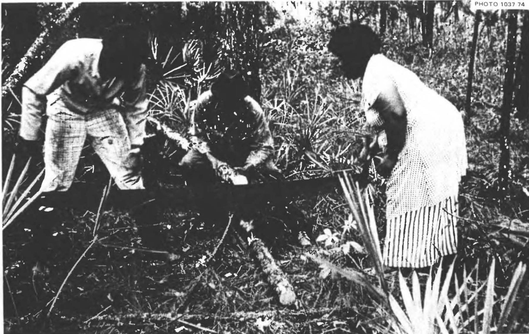
Fig. 5.15. Cutting a small felled tree into one of the specified lengths needed to build pole cribs. Later the cribs were lined with bed sheets and then filled with earth. Instead of following the instructions and pulling long poles to the shelter-building site, where they should have been cut to the desired lengths, this family chose to have the children carry small poles one at a time to the site.
