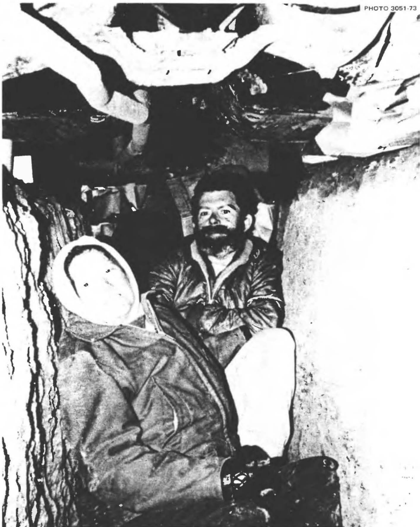
Fig. 6.15. The father (sitting on a box) and the mother in their 40-in.-deep, 28-in.-wide shelter. Enough room remained (occupied by the photographer's leg when this picture was taken) for the small daughter and the family poodle. All of their supplies had been placed under the car.
