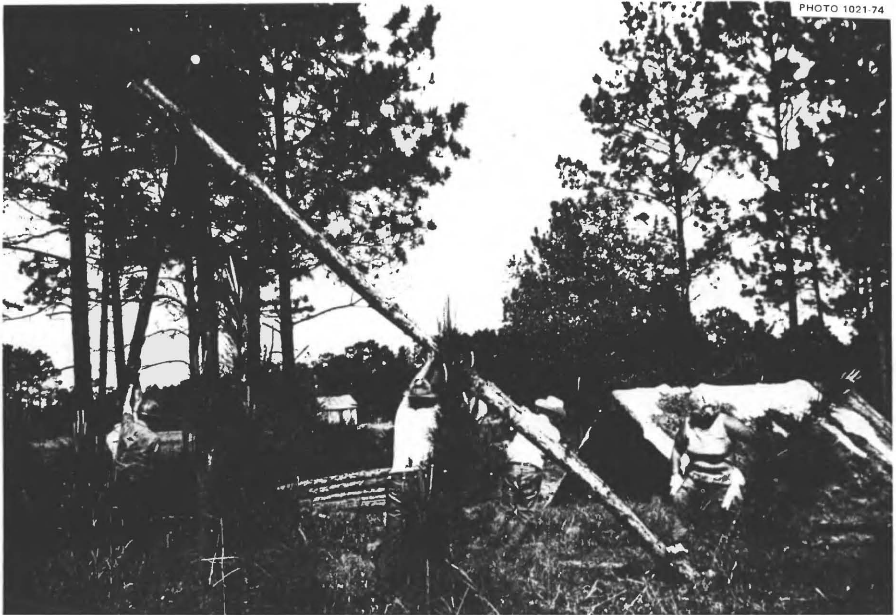
Fig. 5.48. Erecting a tripod made of three 24-ft poles. Kearny's agreement with these mechanized rural Americans specified that they could only use two motor-driven pieces of equipment. To his surprise, they chose to rig a manually operated earth conveyor system, utilizing this tripod, nylon rope, two 5-gallon cans, and pulleys to move earth from the shallow barrow pits to the shelter roof.
