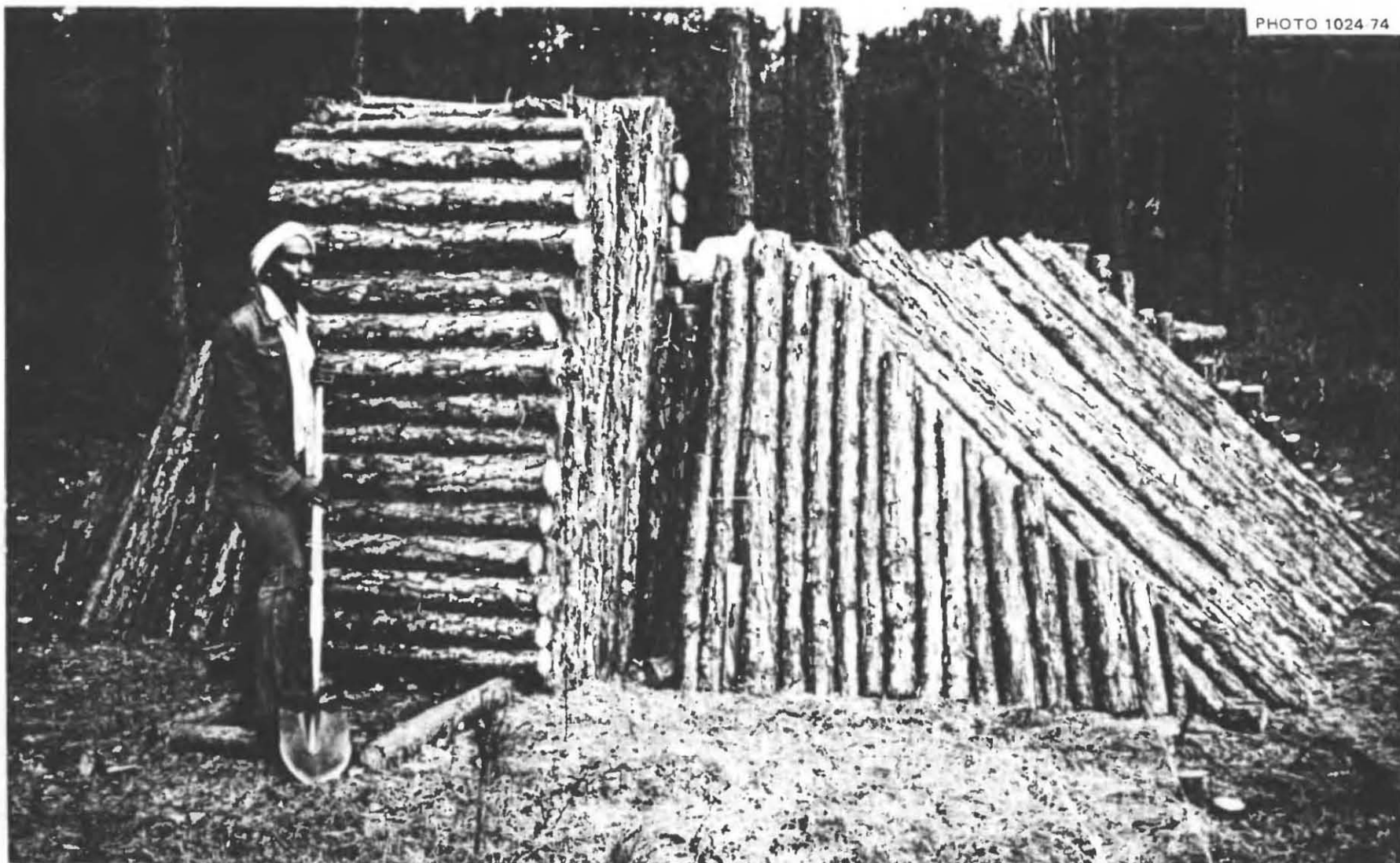
Fig. 5.66. An above-ground Small-Pole Shelter with an interconnected room on each side, beneath 9-ft side-wall poles that slope at 36^\circ . This prototype shelter had 200 sq ft of floor space in its three rooms, was built by a contractor's workmen, and later was covered with a full 2 ft of earth by a backhoe.
