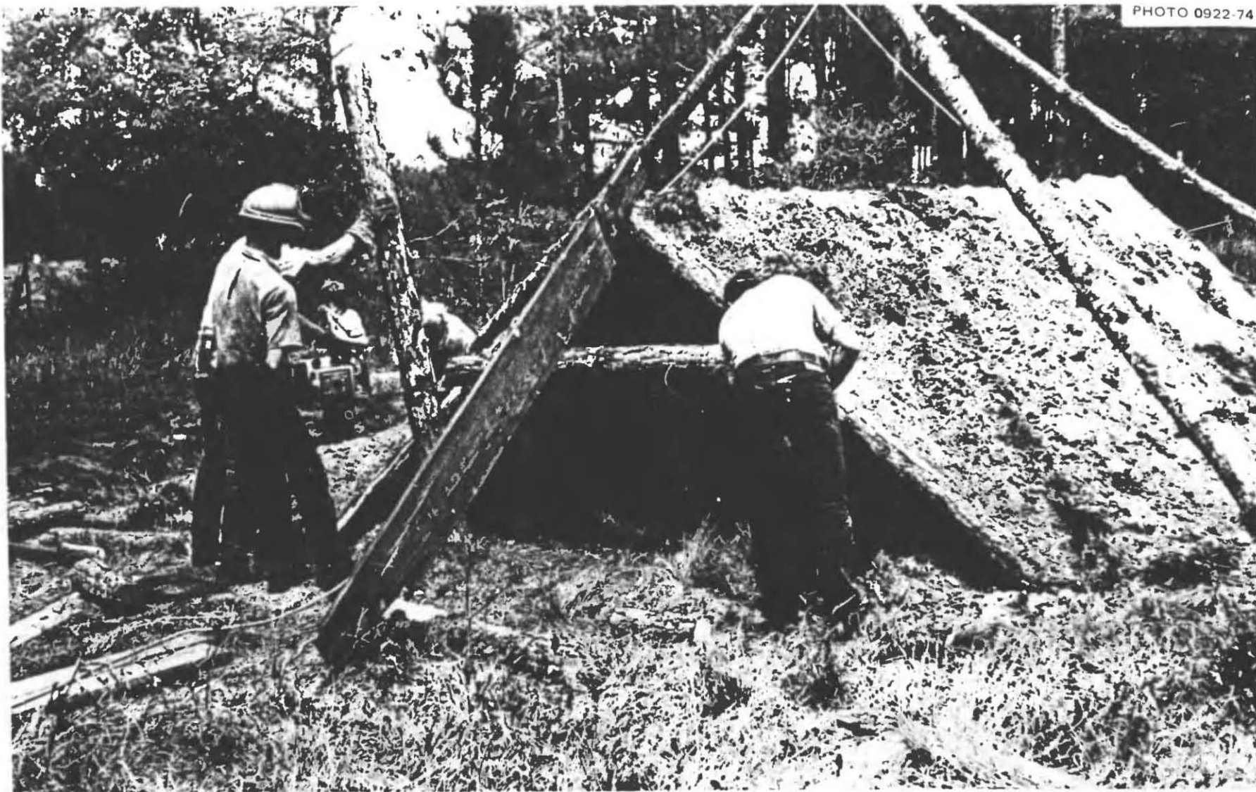
Fig. 5.49. Unnecessary work and delay resulted because these families failed to follow some of the instructions, especially as regards placing earth on the shelter starting from ground level and working upward. While Kearny was going to his car to get some food (the mud prevented his driving his station wagon to this site), the ridge of this shelter shifted lengthwise about 4 in. The builders stopped this move with the board brace pictured and then pulled the whole shelter back into its correct position with a chain and powerful hand-operated winch.
