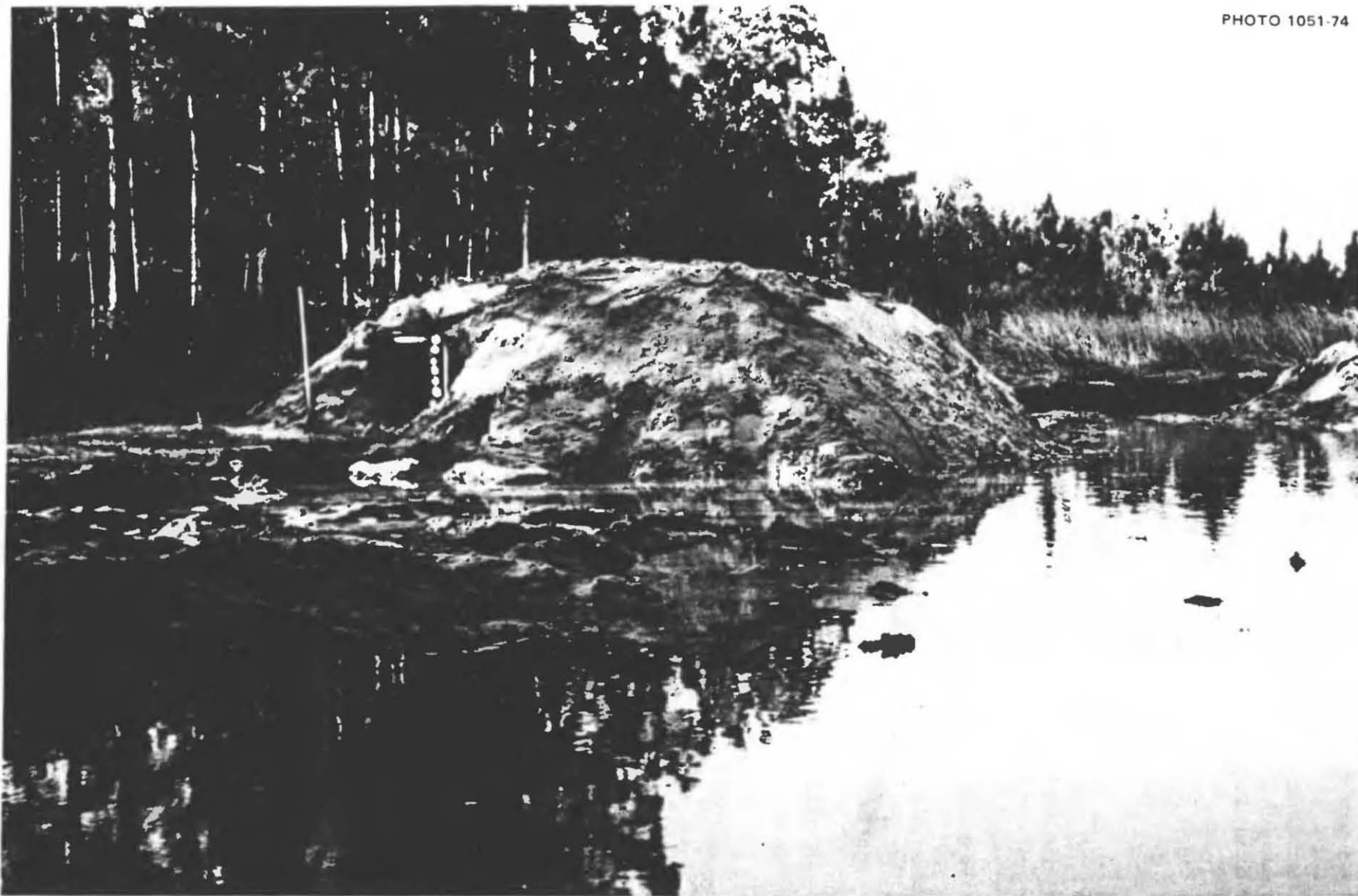
Fig. 5.1. One of the prototype above-ground shelters built by a contractor's laborers in Flagler County, Florida, under the direction of C. H. Kearny, preliminary to the building of shelters by inexperienced family groups. Several prototype shelters of different types were built toward the end of an abnormally dry winter, during a time when a backhoe was able to excavate earth to a depth of about 15 in. without getting stuck too often. The water pictured is in one of the excavations after rains ended the dry spell, showing the normal height of the water table. The water table in most parts of Flagler County is only 1 to 2 ft below the surface.
