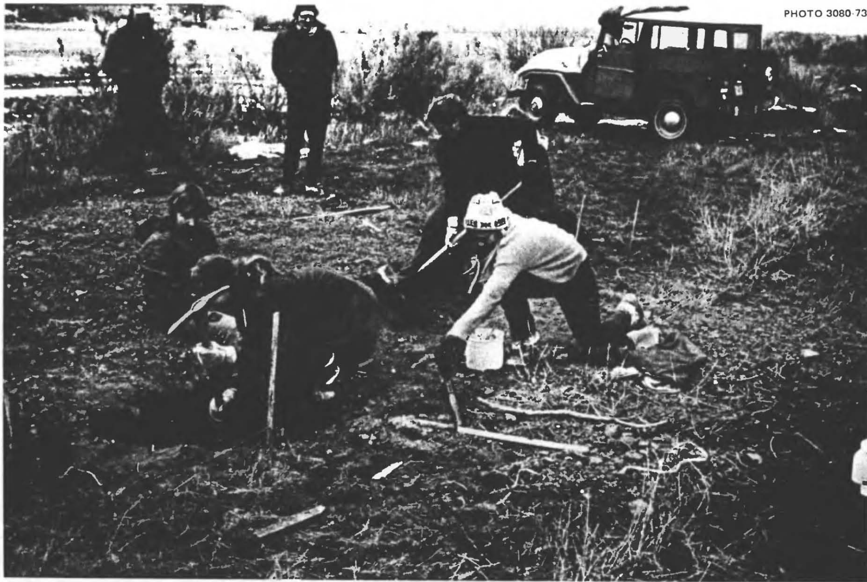
Fig. 2.3. The mother dug inefficiently with her dull shovel by pushing it with her foot. She dug the trench too narrow until it was almost completed – in spite of having read the instructions to the contrary. Until the second day, no member of this family learned to swing their dull old pick properly, by letting one hand slip toward the other as the pick descended. Nor did they know how to use their other tools properly.
