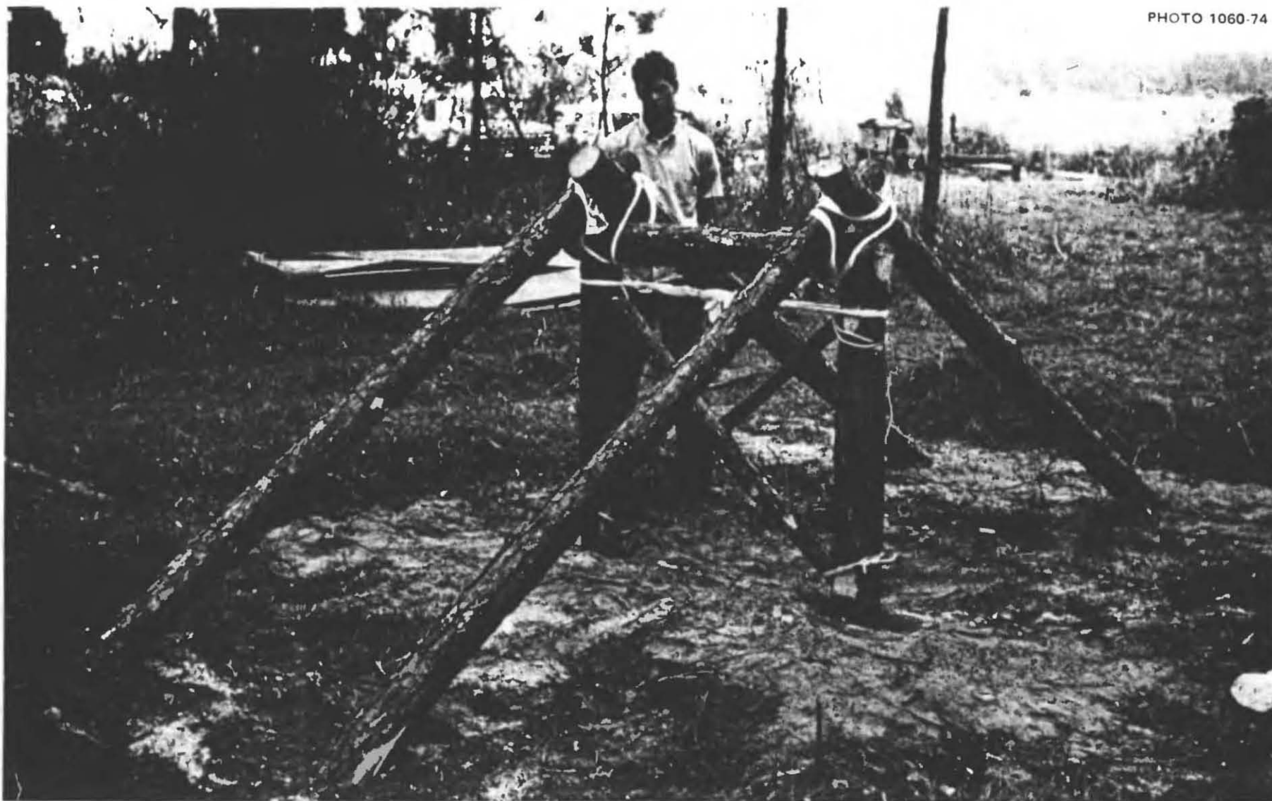
Fig. 5.31. A second prototype of the frame of a Ridge-Pole Shelter, built without using a single nail. Slightly twisted strips of bed sheet, 1 ft wide, were used to hold this simple yet very stable structure together, and three pieces of rope were used to secure the notched cross-braces between the two vertical posts supporting the ridge pole. These vertical posts rested on flattened small areas cut on the upper side of a slightly below-ground footing log. Small poles on the outer side of the vertical posts, just below ground level, prevented any sideward movement of the bottoms of the vertical posts.
