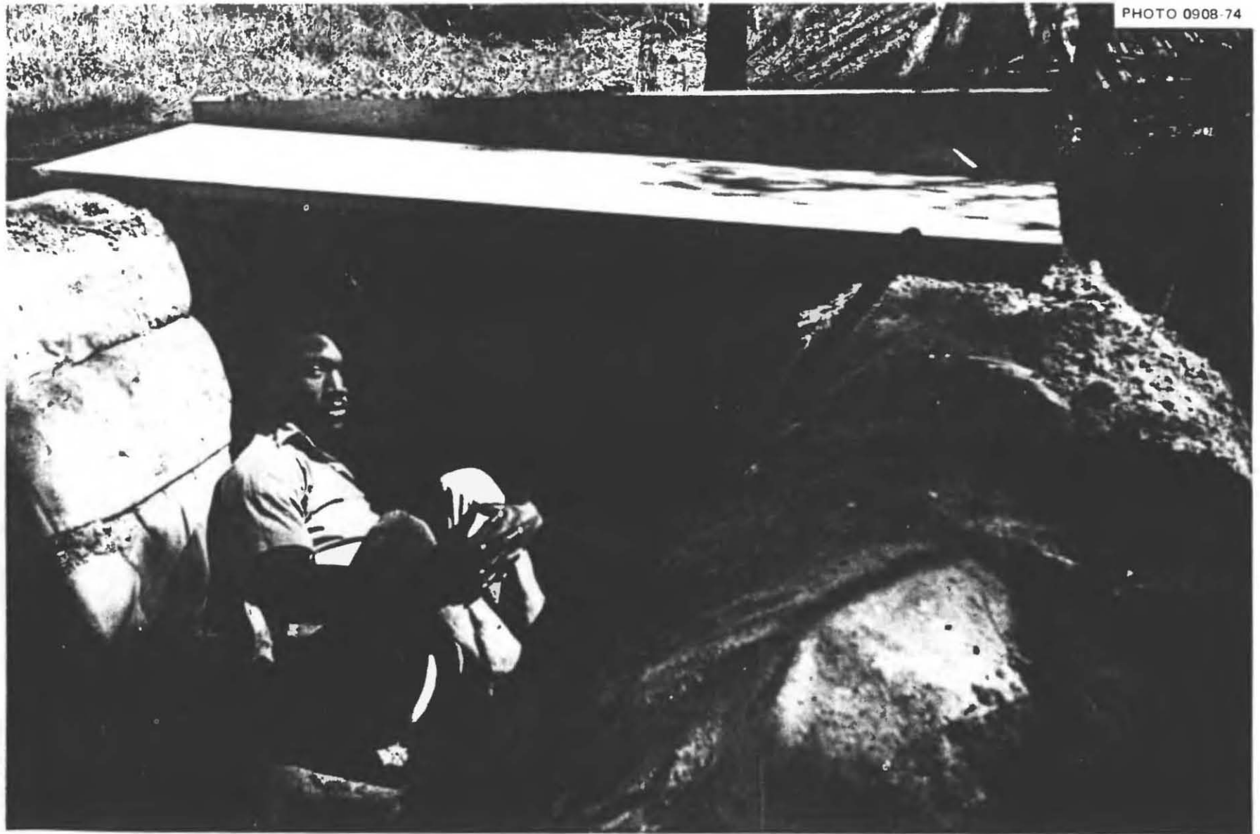
Fig. 5.55. The first of the hollow-core doors used to roof the initial prototype of an above-ground, door-covered shelter using earth-filled rolls for its walls. Since at this time Kearny did not realize that earth-filled rolls made of bed sheets or 4-mil plastic film could be used to form strong and stable vertical walls, these rolls were made sloping inward. This resulted in the free span of the roofing doors being about 5 ft wide. When the single-thickness doors of this roof were loaded with 15 in. of heavy, sandy soil, they broke within 1 to 3 days, although the earth was dry and no rain fell. Humidity, however, was high.
