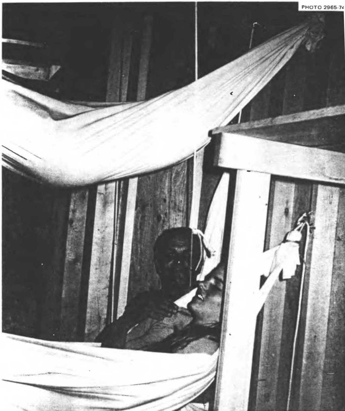
Fig. 4.32. Two Bedsheet Hammocks, one above the other, slung in the entrance end of a lumber version of a Russian-type Small-Pole Shelter. On the right is seen the end of one side of the typical Russian-style benches with overhead boardbunks. The Russian sitting-sleeping system is a "hot-bunk" system that enables only one-third of the occupants to lie down at the same time.
