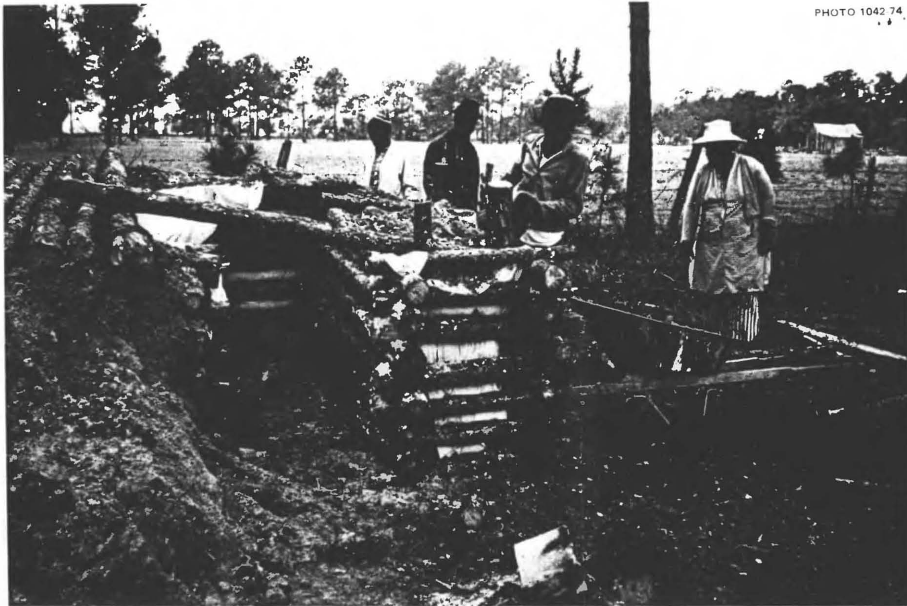
Fig. 5.19. One of the two entryways of this Crib-Walled-Shelter, showing a sheet-lined, earth-filled end crib almost filled with earth. The two entryways, one at each end of the shelter, faced in opposite directions, assuring adequate cooling except in very still, hot, humid weather.
