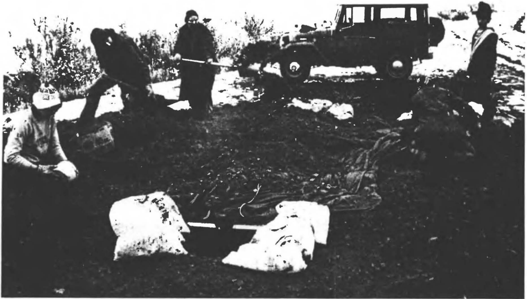
Fig. 2.10. Covering the water-shedding "buried roof." This family used a tent, due to a desire to save their shower curtains and most of their plastic table cloths, etc.
