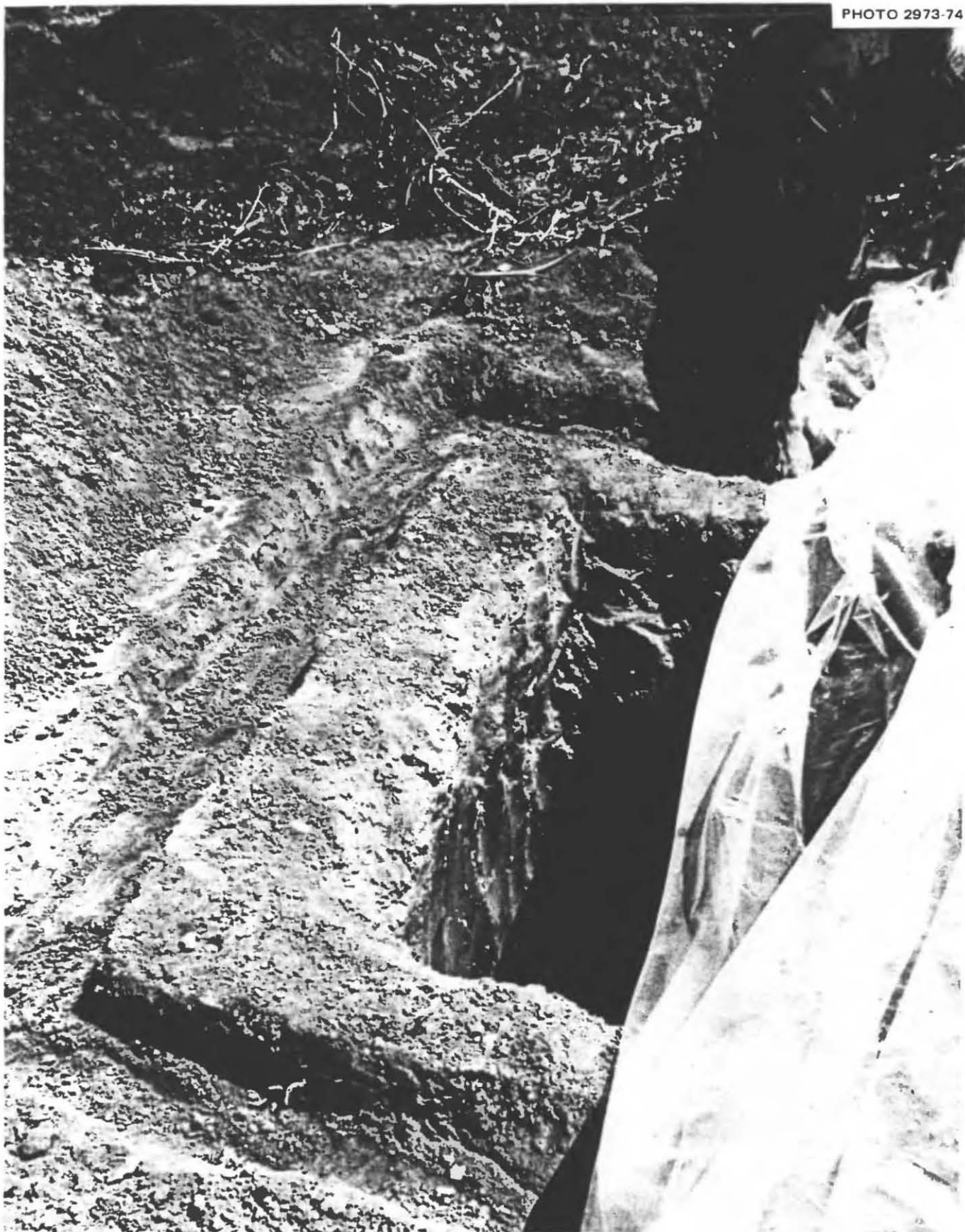
Fig. 4.34. Placing a sheet of 4-mil polyethylene in a 120-gallon water-storage pit. Unlike previous water-storage pits dug and tested by Kearny, this pit was not first lined with cloth or other material to keep sharp roots, etc., from puncturing the waterproofing plastic. All root ends were merely cut off with a knife. The edges of the plastic were folded into the small side trenches, and then held by packed earth. Six days after being filled, no leaks had developed.
