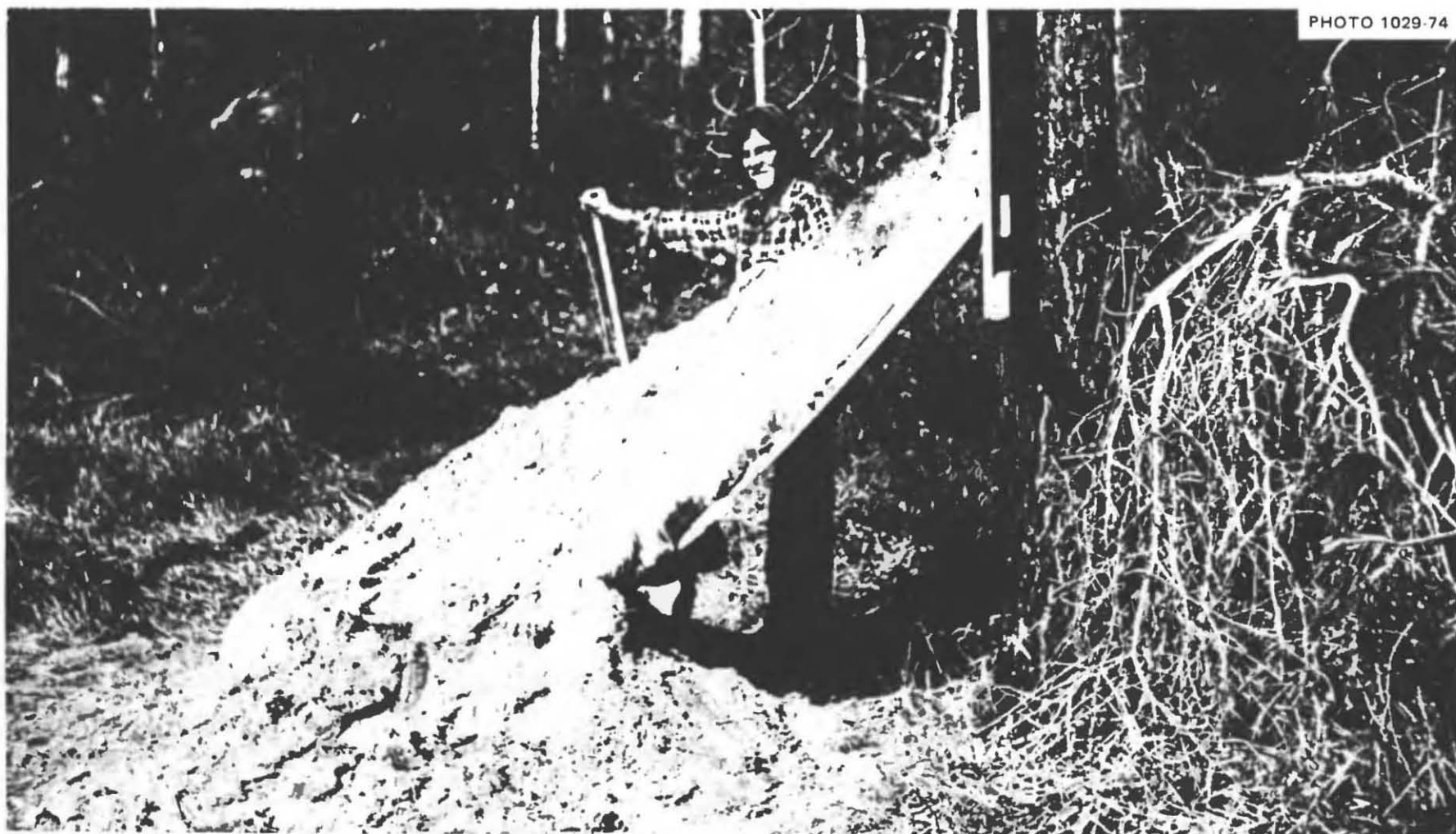
Fig. 5.65. A single hollow-core door simulating a section of the roof of a Tilt-Up Door Shelter. The unnecessary shelf had been removed; an earth cover approximately equal to the specified weight of earth for the double-thickness roof doors of the DCPA shelter was positioned. The door had been covered with 4-mil polyethylene, and earth-filled rolls were placed along both its sides. These rolls made it possible to place steep-sided earth cover on the door.
