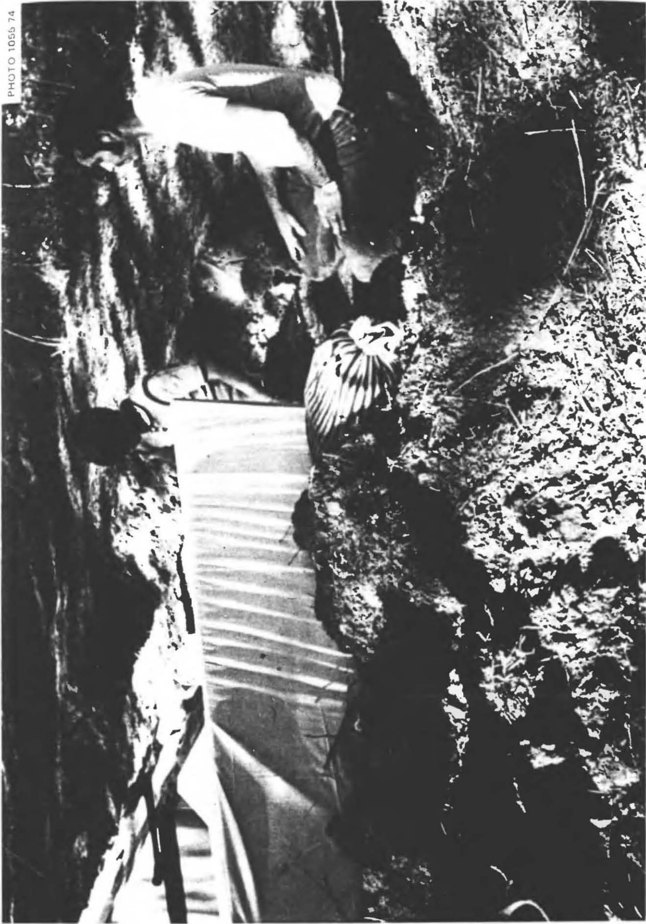
Fig 5.6. Starting to make the lowermost roll to form the wall at one end of the shelter. The striped sandbag is made of a child's pillow case, one of several used to form the outside supports of one entryway wall.
