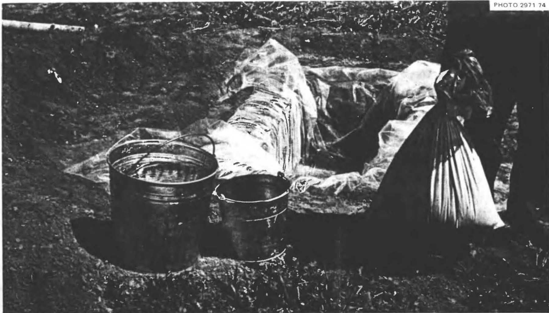
Fig. 4.35. The 120-gallon water storage pit of thin plastic being filled. This pit was later covered with boards, over which thin plastic was placed, and then earth was mounded over the boards, about 6 in. deep in the center. Next, a waterproof, outward-sloping "buried roof" of the plastic was laid on top of the mounded earth. Finally, about 4 in. of earth was mounded on top of the buried roof.
