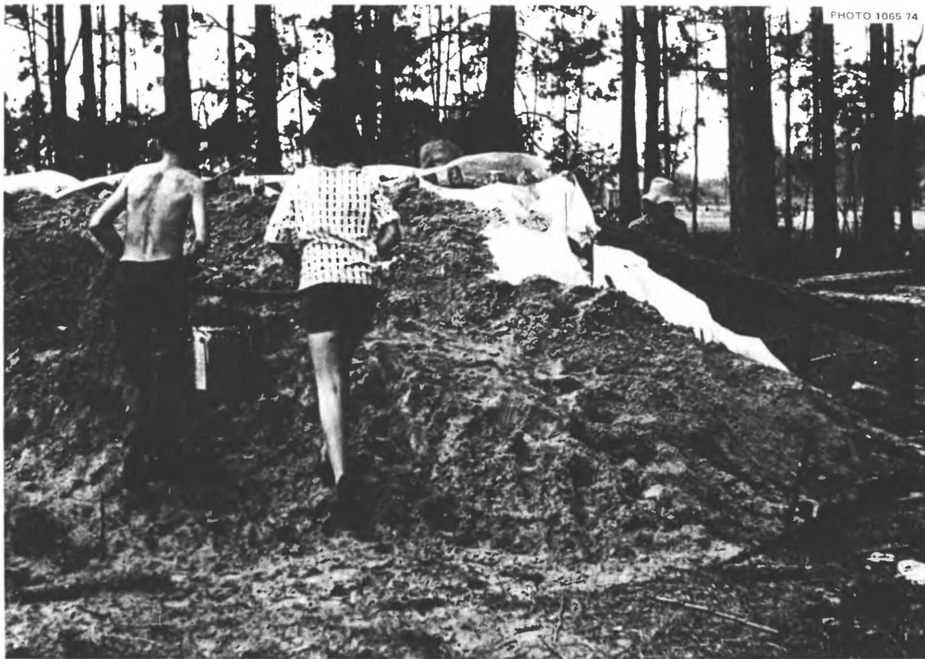
Fig. 5.36. Two teenagers carrying earth in a 5-gallon bucket, from one of the shallow barrow pits. These builders found that carrying earth in this manner enabled even children to move earth effectively, all the way to the top of the shelter.
