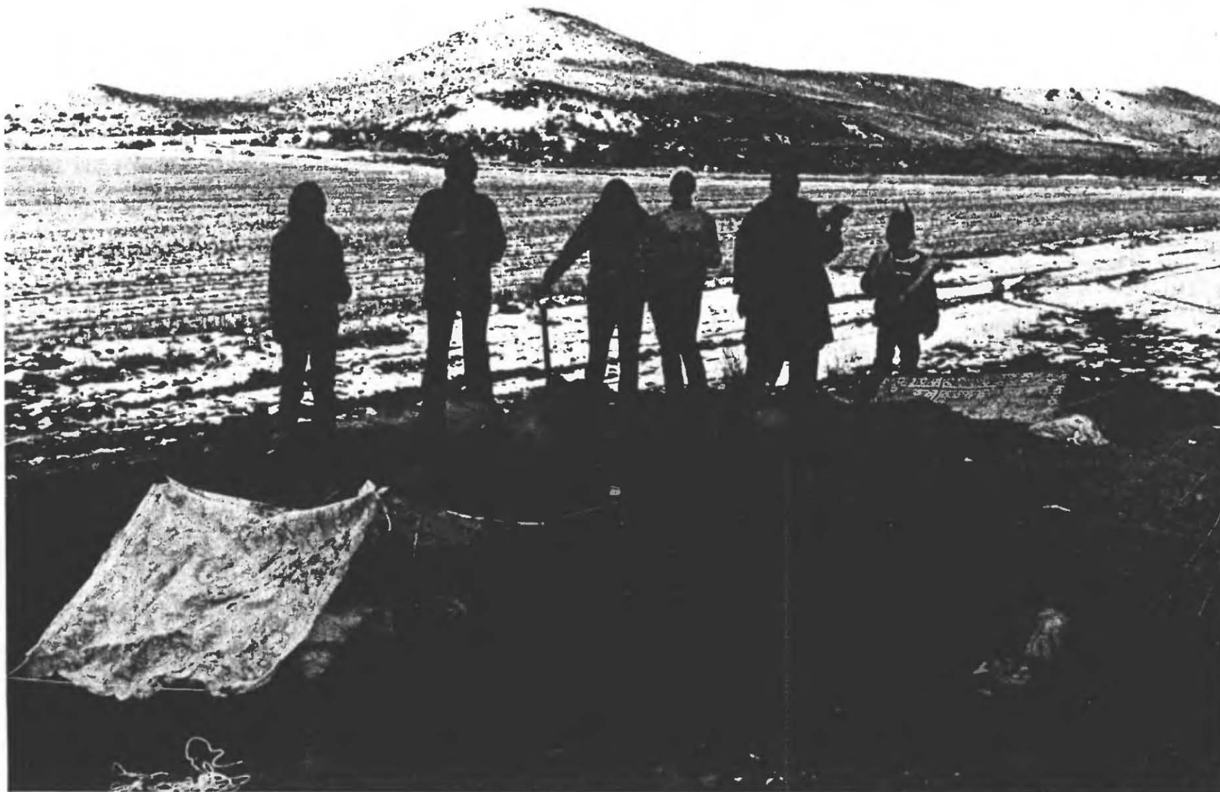
Fig. 2.11. Completed Door-Covered Trench Shelter, with canopies made of plastic tablecloths inexpertly rigged over the two openings.
