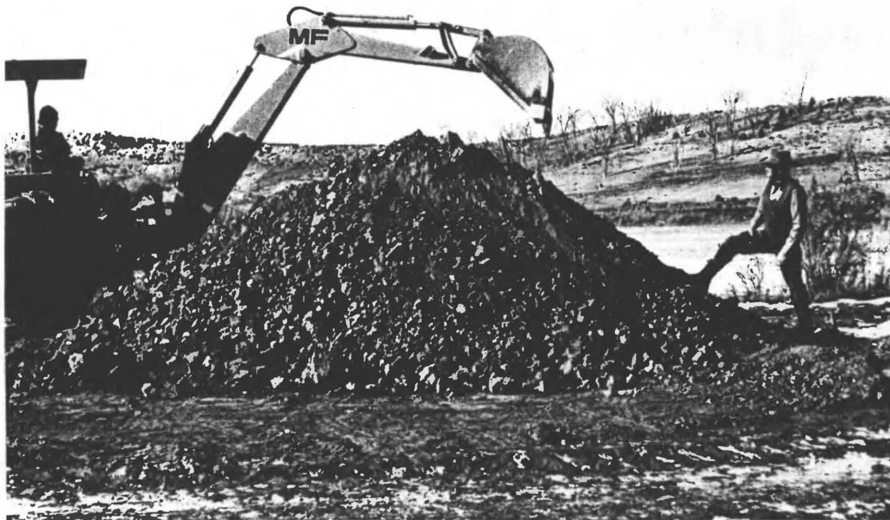
Fig. 3.1. Six and one-half feet of earth piled on December 1 over the 6-door Door-Covered Trench Shelter built by the manless family on November 24 and 25, 1973.
