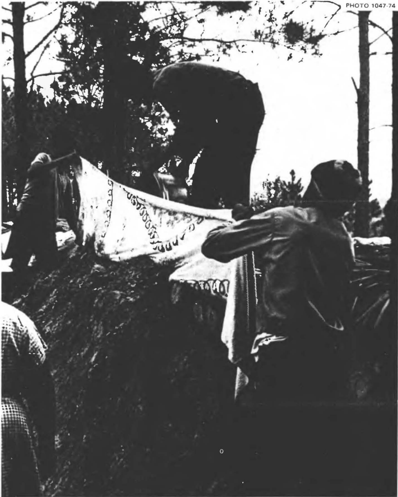
Fig. 5.22. Using an old bedspread to form an earth-filled roll along an upper edge of the essentially flat shelter roof of poles. The father is pouring earth out of a large bucket. These rolls made it possible to increase the stability of the earth covering around the edges of the roof, and also prevented heavy rains from washing any appreciable amount of shielding earth off the shelter roof.
