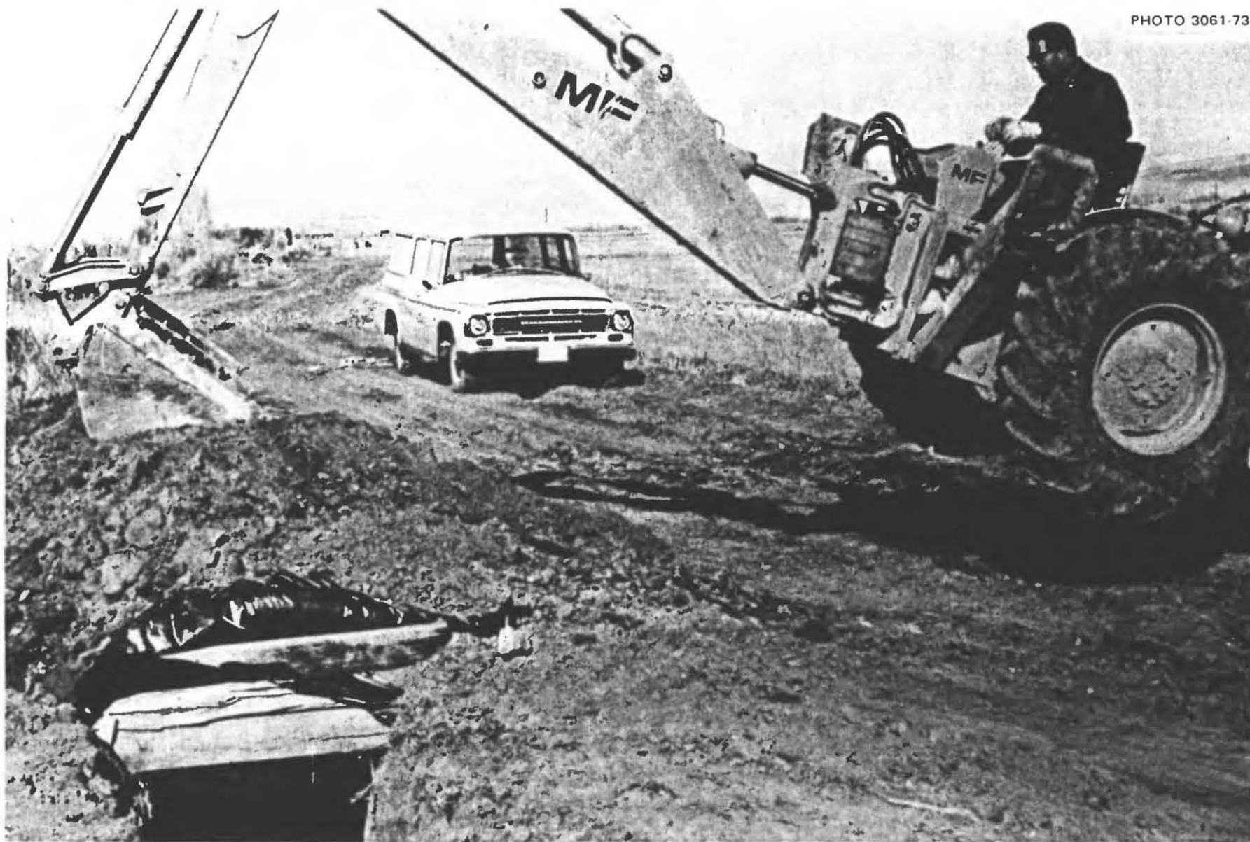
Fig. 3.13. Stressing the Tarp-Roofed Trench Shelter, a 6-ton backhoe, supported only by its buckets, pressed down repeatedly with its front bucket on a 62-in.-deep mound of loose earth. The mounding of loose earth caused the tarp to bow downward (sag) into a catenary curve. The compaction caused the tarp to stretch, resulting in an increase of the maximum sag from 8 to 14 in.
