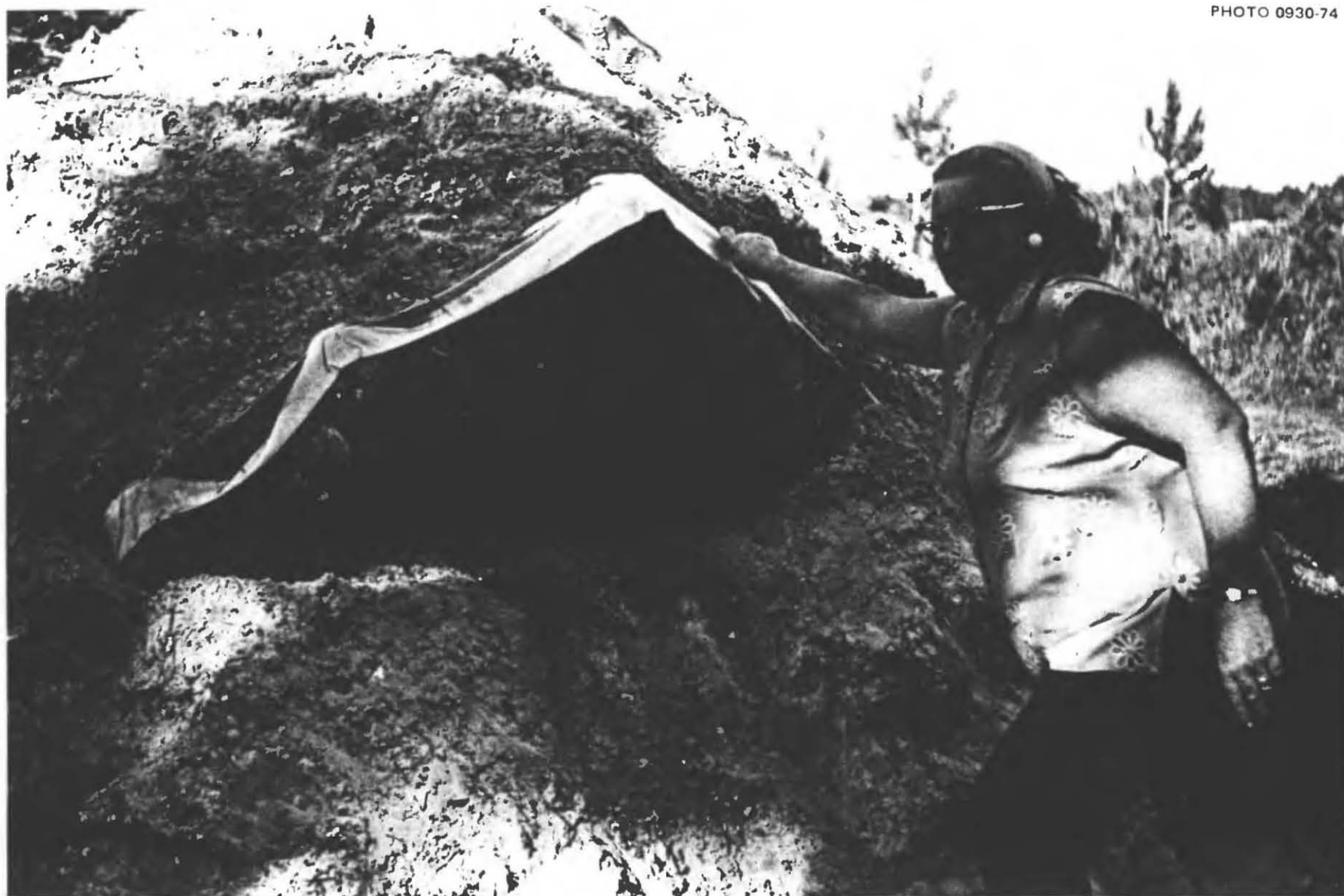
Fig. 5.50. The simplified, but not as protective, ventilation opening constructed in what had been the end of the shelter toward which the skewing movement occurred. Seven-foot poles were placed on the roof poles, parallel to the ridge board and extending 3 ft beyond the outermost wall poles. Those 7-ft poles formed the overhanging gable shown in this photo. Later, the earth cover was thickened.
