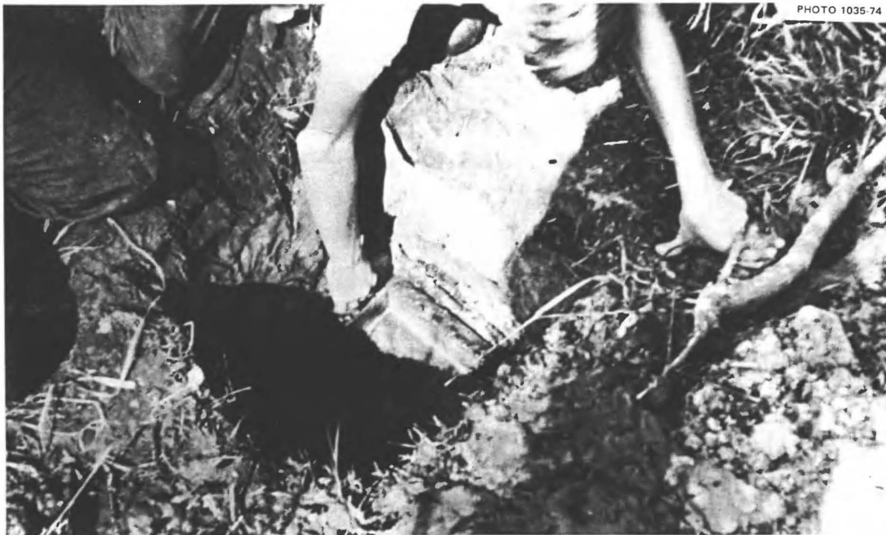
Fig. 5.70. A shallow well for drinking water, dug into the free-flowing sand below the water table. Note the rectangular board shoring, which was forced downward as the free-flowing sand was dug out from inside and below this shoring frame. Twigs and leaves were stuffed in behind the frame, to help check the inward flow of sand, that otherwise would have led to the collapse of the sides of this well. Without instructions, average Americans would not be able to dig a well inside their shelter, from which they could dip water repeatedly without causing disastrous caving.
