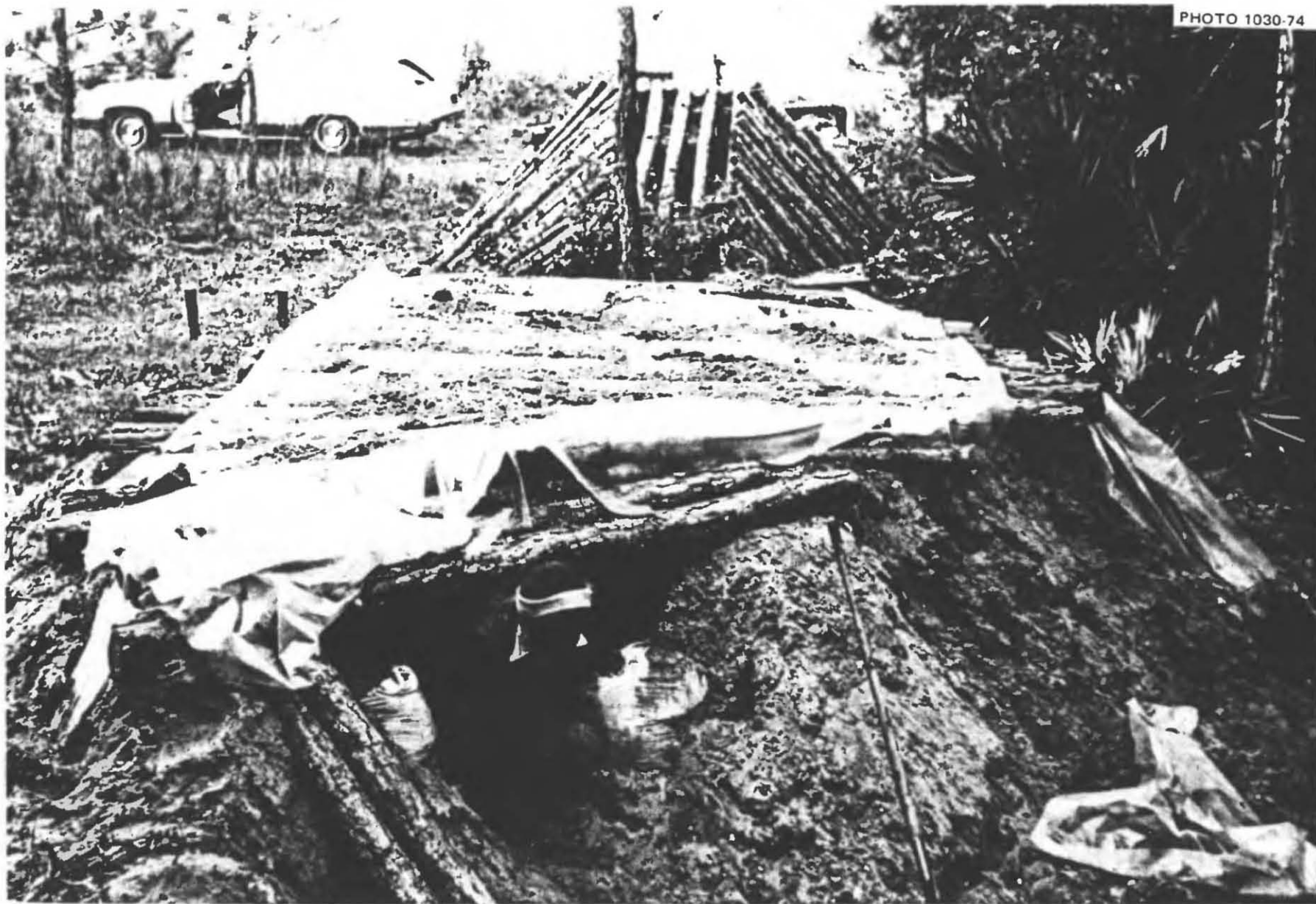
Fig. 5.57. The same shelter after being roofed with substantial pine poles placed on the walls made of undamaged rolls. Later, 2 ft of earth was mounded over these roof poles. At the time this shelter was completely demolished, almost one month later, the sheet-covered rolls were still in satisfactory condition. However, where black organic matter was in contact with cotton sheets, the fabric was beginning to rot.
