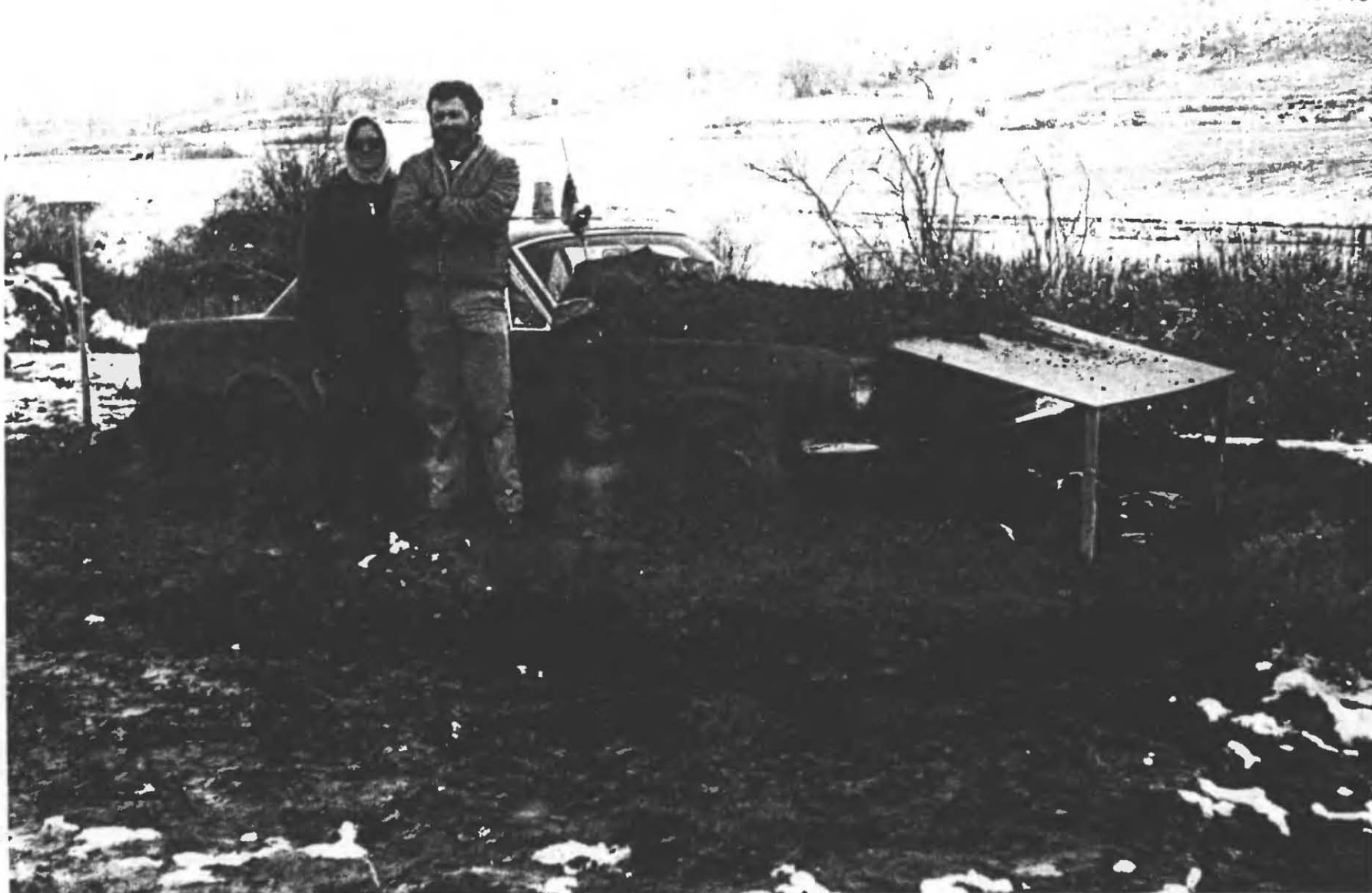
Fig. 6.14. The Car-Over-Trench Shelter was completed at 4:15 PM on the second day. The father did about 95% of the work; 14 hours and 27 minutes were spent working at the site. This family did not win the bonus for completion within 24 hours from the time work began.
