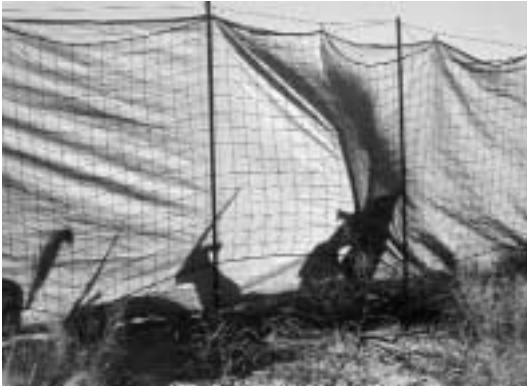
Plastic sheeting reinforced with a net. Photo: J. du P. Bothma.
